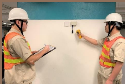
Installation of IoT sensors at carpark
