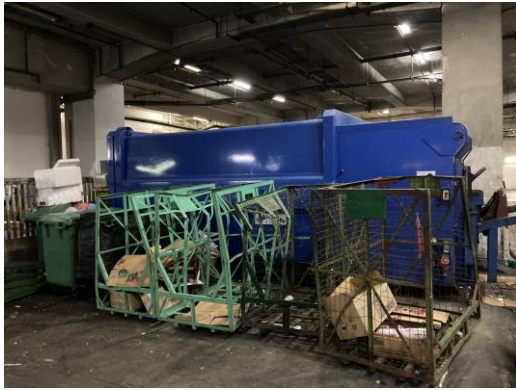
Waste compactors located at the central refuse collection and storage point of some commercial buildings.
