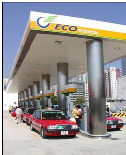
Figure 5. LPG Filling Station
