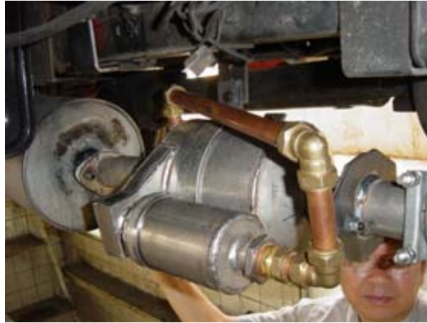
Figure 4. The installed particulate removal device
