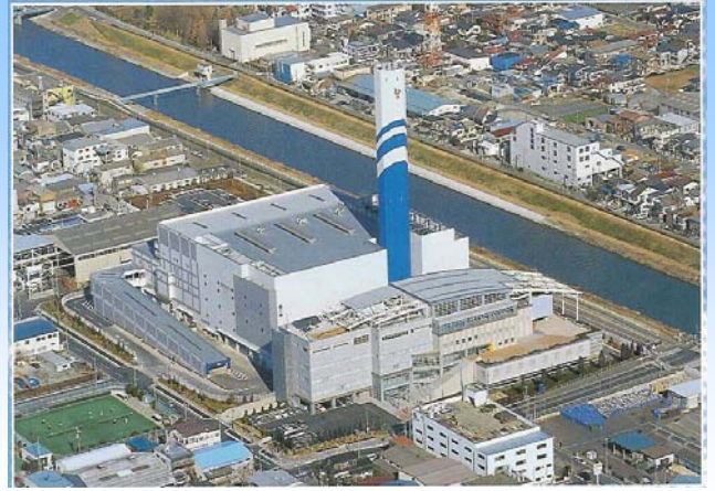
Gasification and Ash Melting Plant
