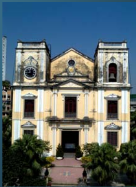
St. Lawrence's Church – Originally established before 1563
